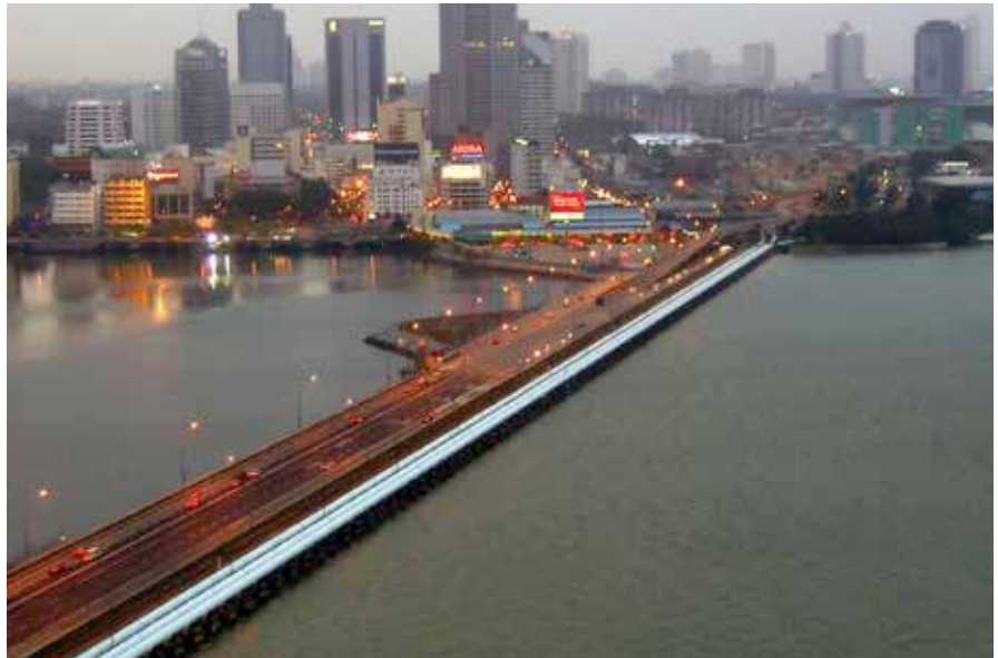
Singapore-Johor causeway is not only a bridge that connects the two countries, along it also lies the pipes for the water Malaysia supplies to Singapore. Image: Calvin Teo, CC BY-SA 3.0 via Wikimedia Commons
