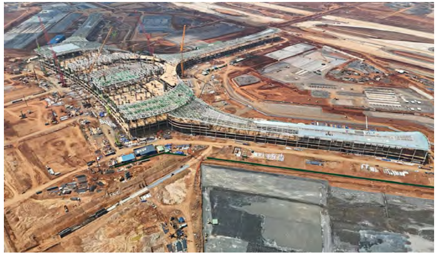
Expansive aerial shot of a construction site with cranes and building foundations in Dong Nai, Vietnam. Image: Toàn BDS/Pexels
