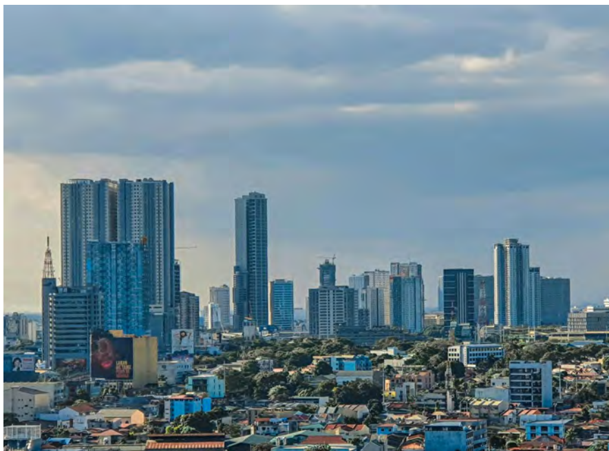
Construction projects in Quezon City, Metro Manila, Philippines. Image: Rey Melvin Caraan/Unsplash
